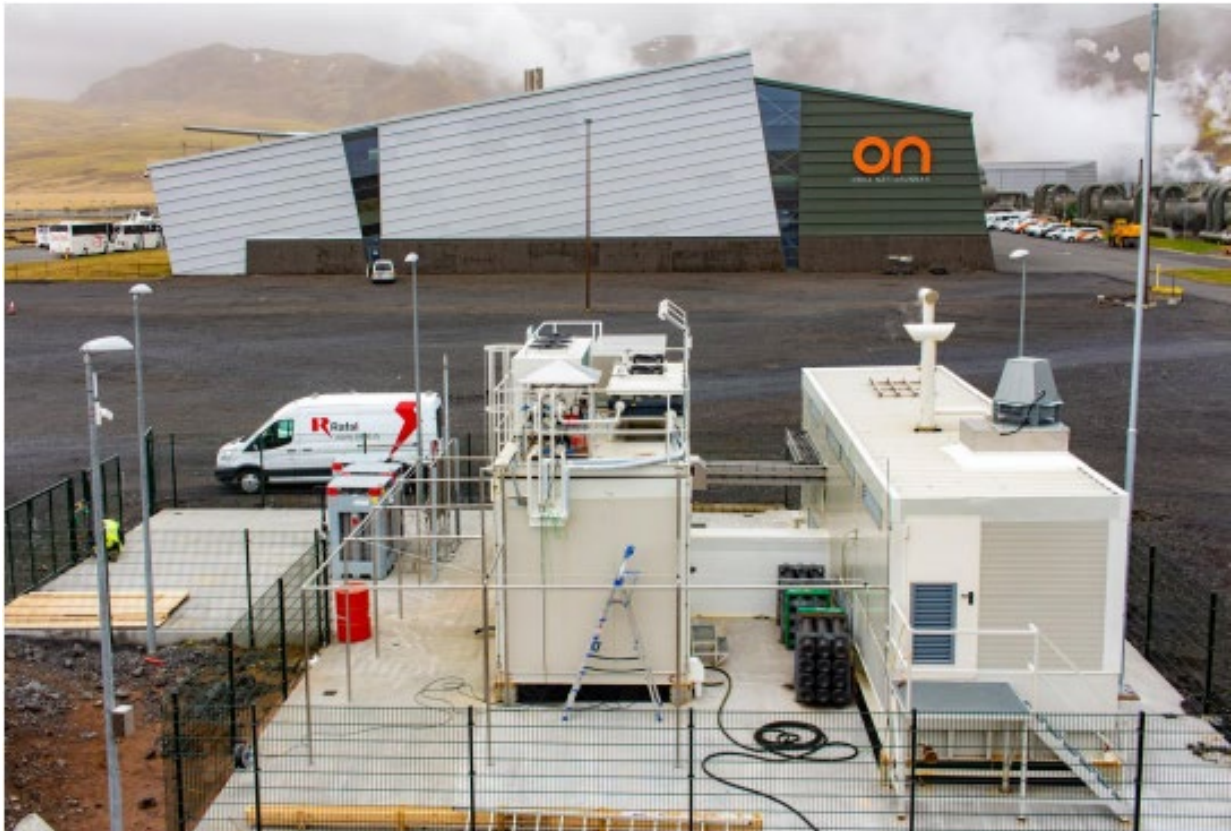
Figure 11.5. Hydrogen pilot plant at Hellisheiði (Source: ON power).
