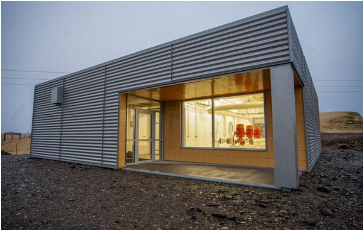
Figure 11.7. Pumping station for the new geothermal district heating system in Hornafjörður municipality, SE-Iceland.
