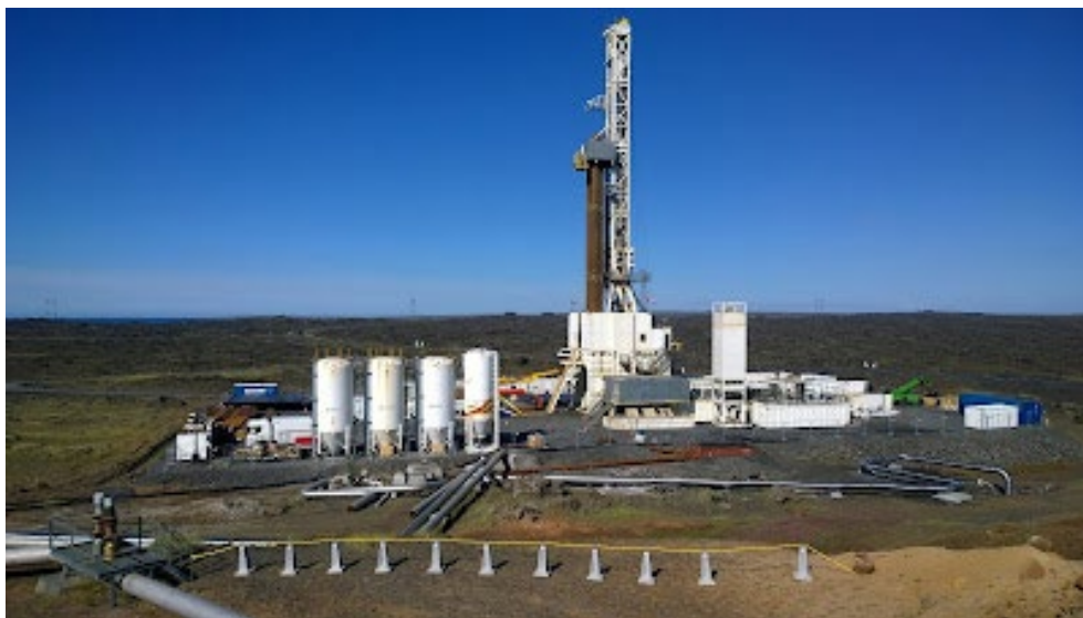
Figure 11.8: IDDP-2 in the process of drilling (Source: HS Orka).
