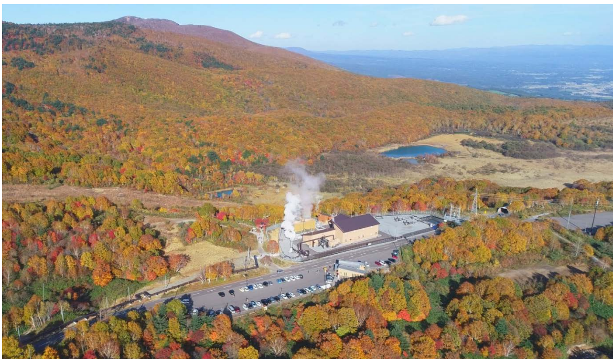
Figure 13.2 Matsuo-Hachimantai Geothermal Power Plant (7,499kW, single flash, operational 29 January 2019). Photo by Iwate Geothermal Power Co., Ltd.
