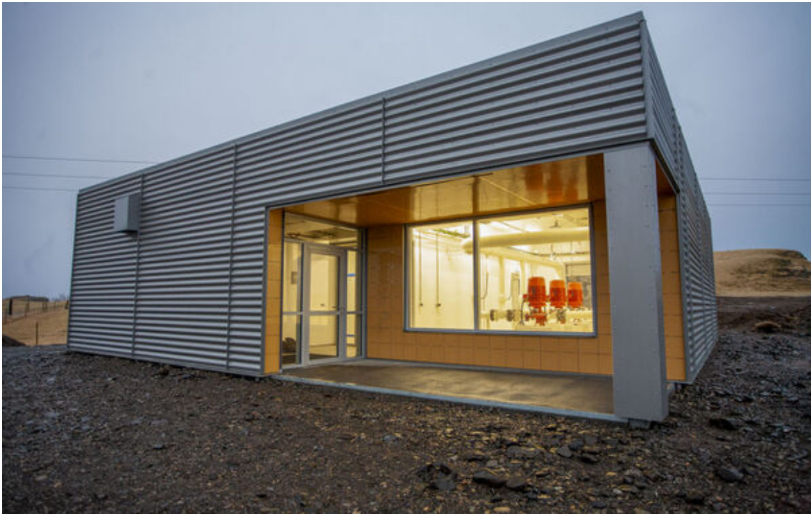
Figure 11.7. Pumping station for the new geothermal district heating system in Hornafjörður municipality, SE-Iceland.
