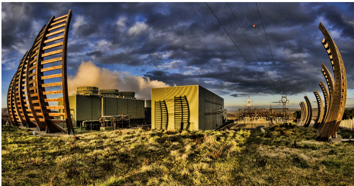
Figure 12-1: Nuova San Martino Power Plant
