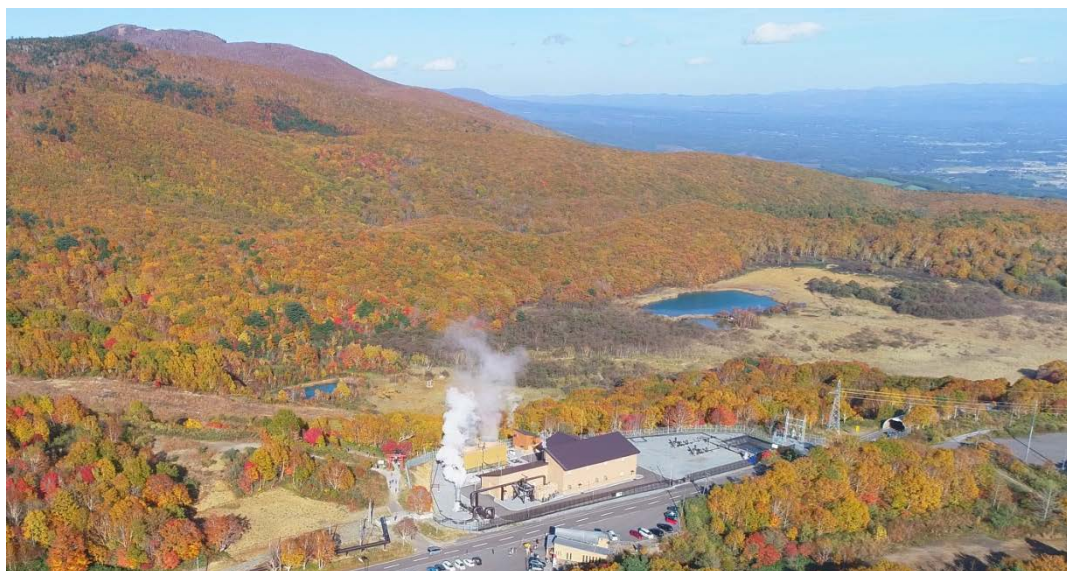
Figure 13-4 Matsuo-Hachimantai Geothermal Power Plant (7,499kW, single flash, operational 29 January 2019). Photo Iwate Geothermal Power Co., Ltd.
