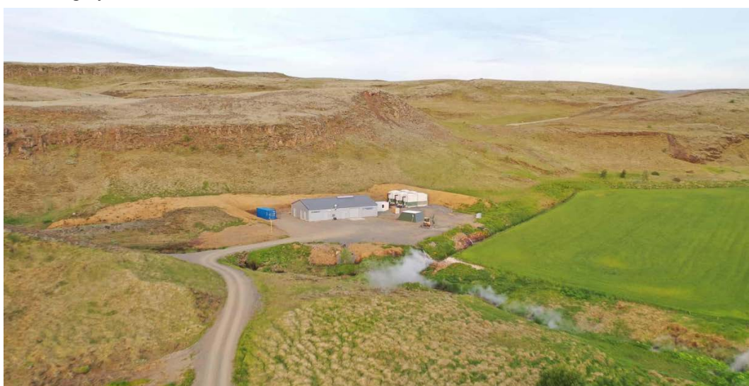
Figure 11-4. Geothermal plant in Flúðir, South Iceland (Varmaorka).
