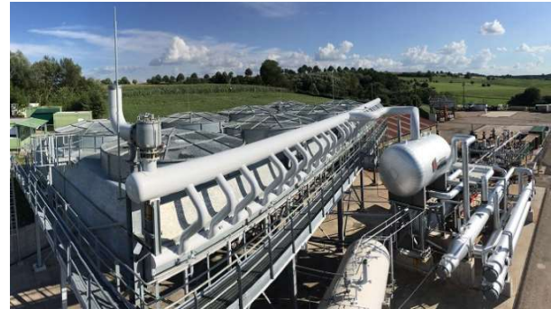
Figure 5: Aerial view of the Soultz-sous-Forêts binary plant (source: GEIE EMC).
