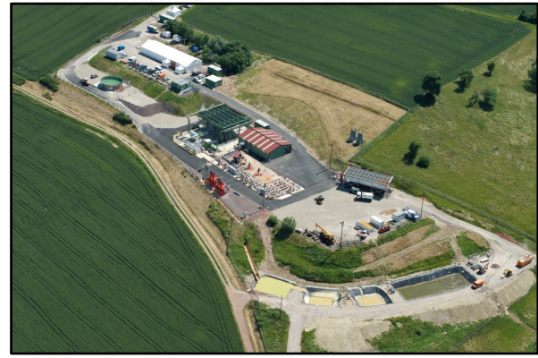
Figure 2: Aerial picture of the new revamped plant in Soultz-sous-Forêts (Courtesy of ES Géothermie)
