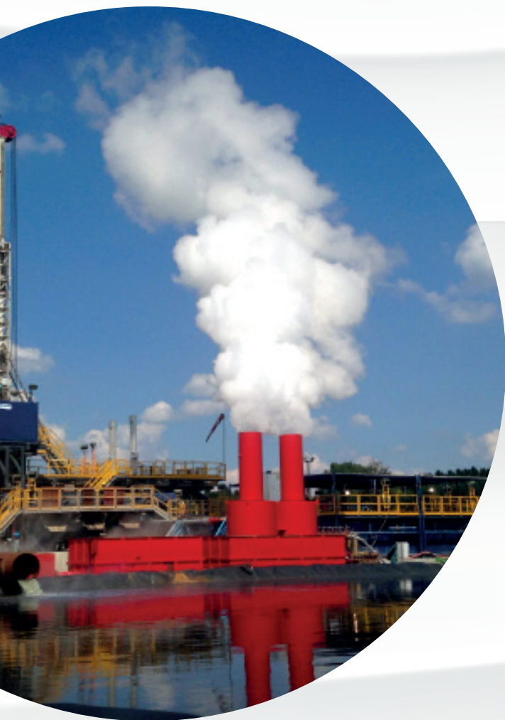
Geothermal power plant in Rittershoffen (Alsace)
